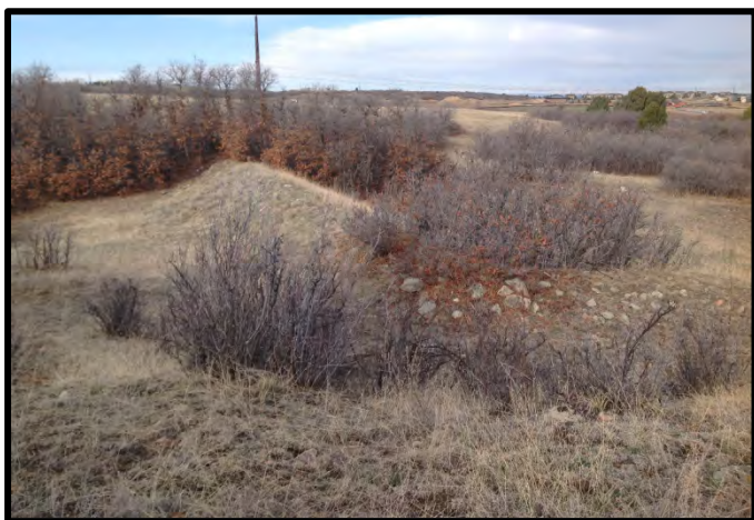
Figure 3. Flood-control dam with spillway in the foreground.
