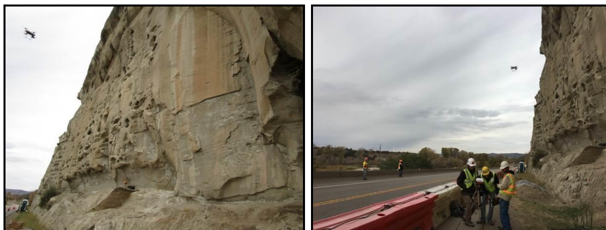
Figure 3. CDOT's drone taking a photo of Alpine's excavation block.
